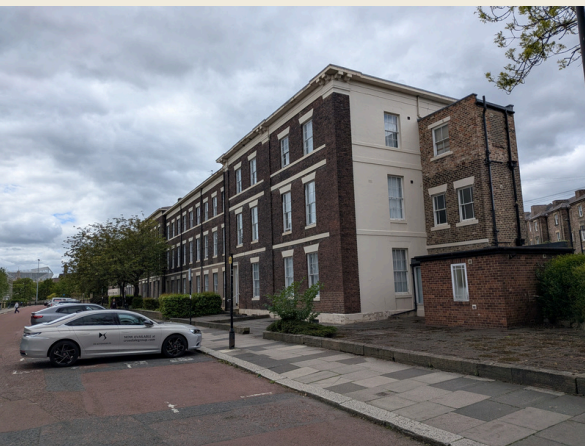
VIEW OF 47-49 LOOKING WEST
