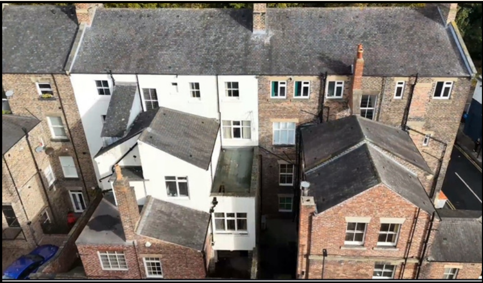
AERIAL VIEW OF REAR ELEVATION
